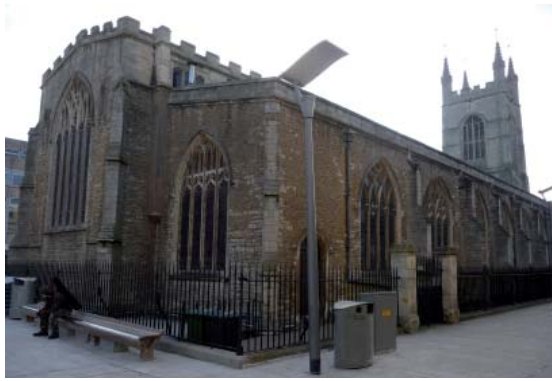
Historic railings and new street furniture
