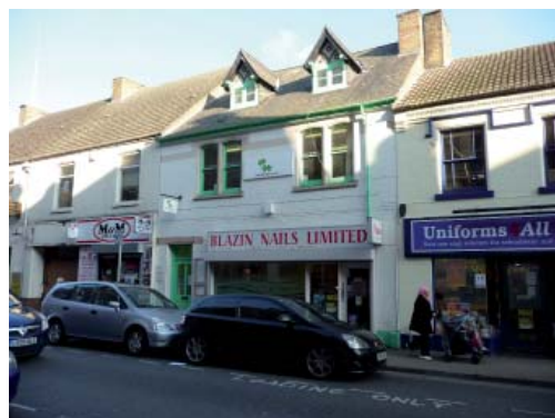
Brick and slate C19 buildings, Park Road with some modern replacement materials
