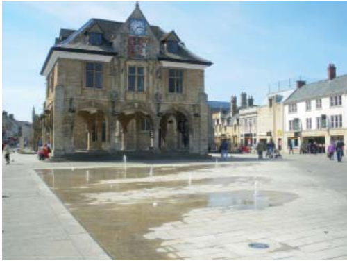
Public realm improvements, Cathedral Square
